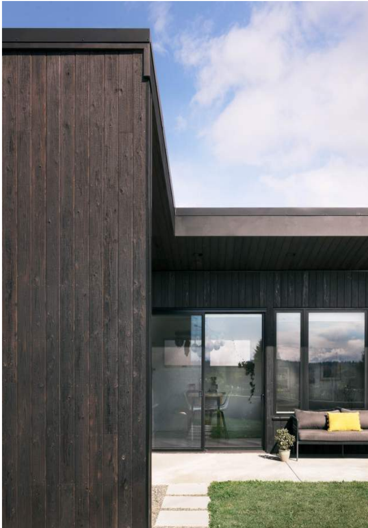
The couple chose shou sugi ban siding, with an extra treatment to meet stringent fire codes.
