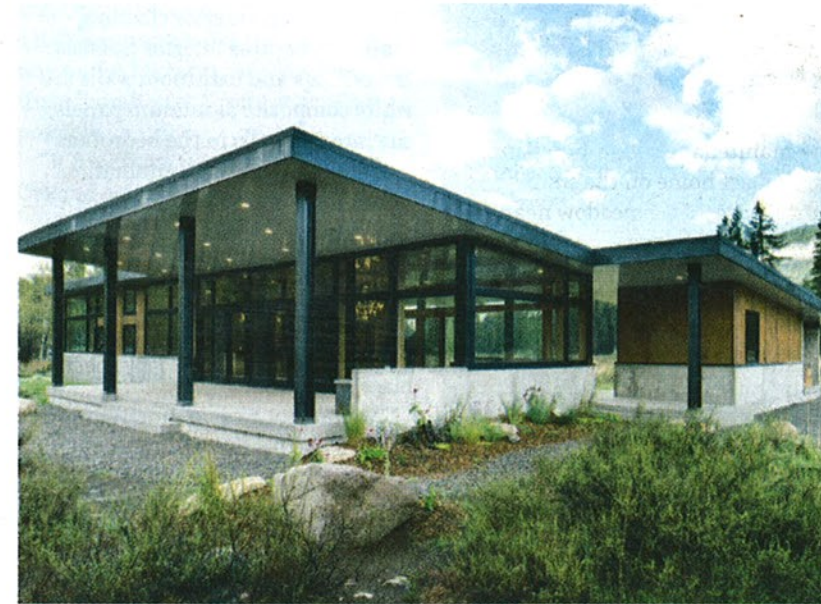
The home is designed to be unobtrusive in its surroundings. PHOTO COURTESY CAST ARCHITECTURE
